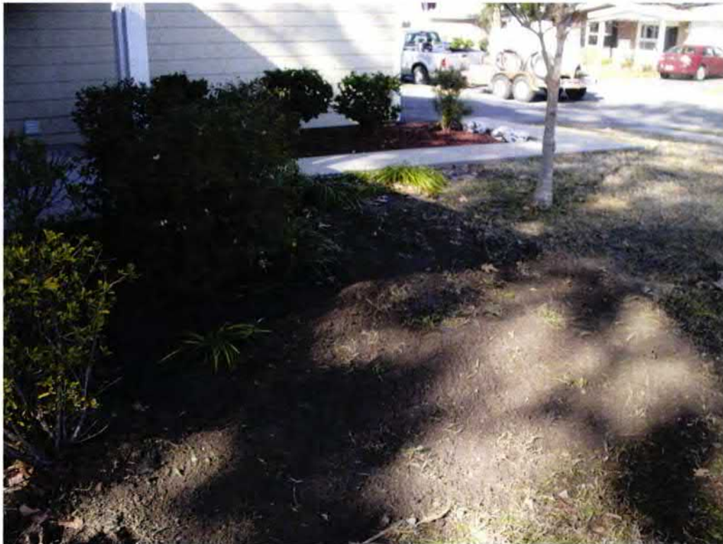
Picture 4: Site after completion of work.
